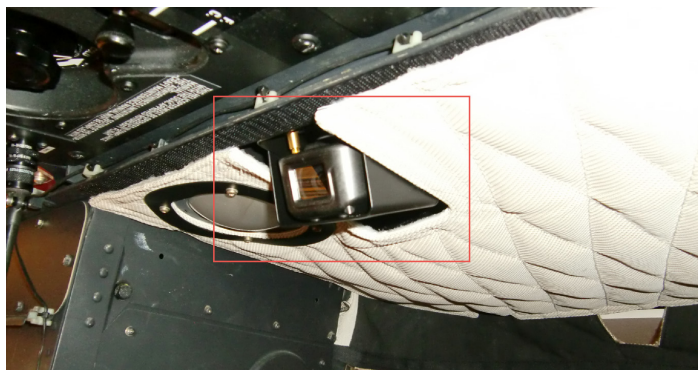
INSTALLED IN AIRCRAFT (COCKPIT CEILING)
